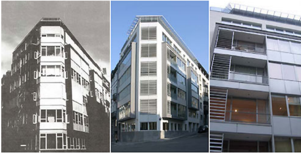
Figure 2 : 44, avenue de l'association (arch. Roose and partners)
